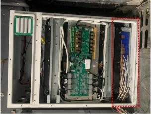
Figure 10b. Internal view of initiating module.
